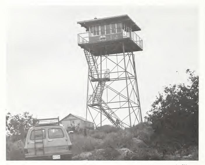
Figure 167. Saddle Mountain lookout, a CL-100 series cab on a Aermotor MC-24 tower, on the Gila.
